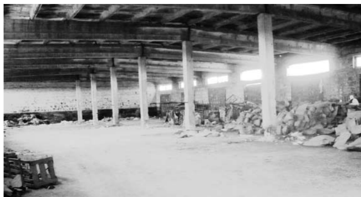
Figure 5: Interior of the building of the big storage. Author: Z. Honzajková
