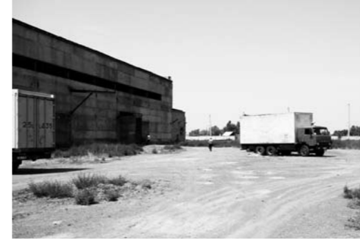
View of the commercially used facility. The pesticide storage rooms are located at the end of the hall.
