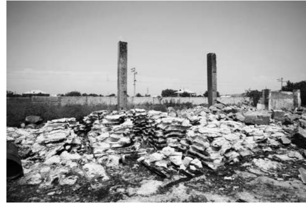
Demolished building (look from the „inside“), where numerous bags probably containing pesticides were found. No samples were taken here.
