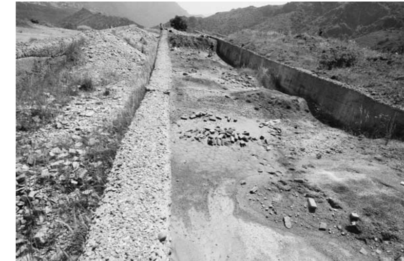
Concrete enclosures containing copper production waste at the dumpsite close to the village Lernahank.
