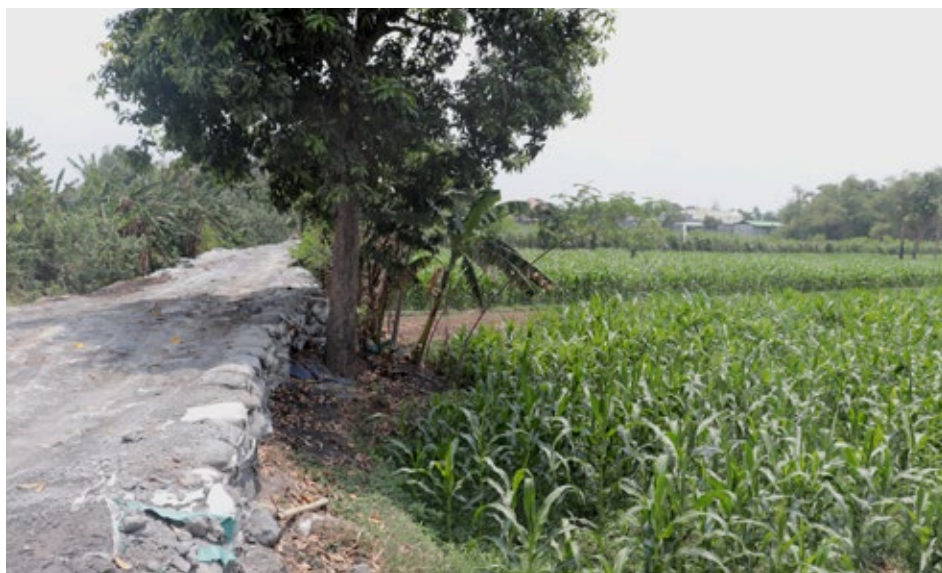
Photo 29: Rice crop field near Sidokampir, where all samples of soil, dust from the road and rice crop were taken in the years 2018 and 2019 (see Table 1). The road was built from ash in big bags, as is the usual practice in Kendalsari and Sidokampir. Photo: Jindrich Petrlik, November 1, 2019.
