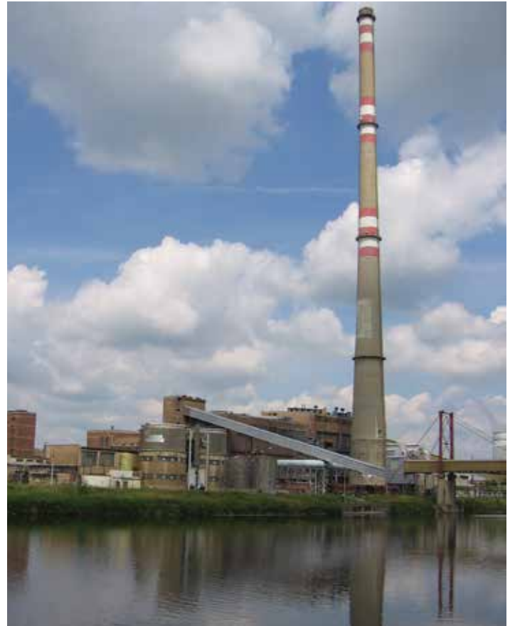
The chlor-alkali plant Spolana in Neratovice lies on the River Labe.
