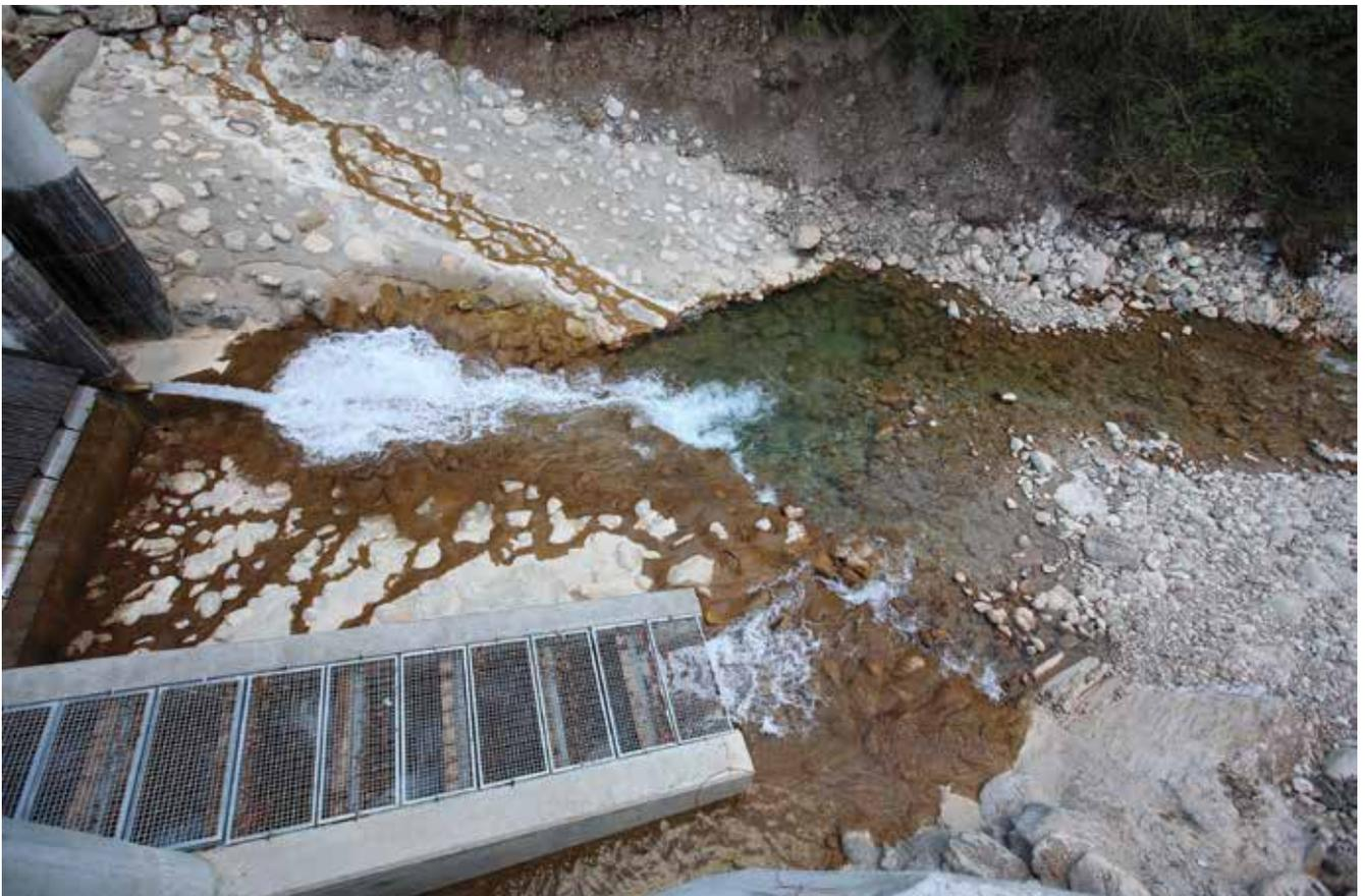
*Fish ladders are built according to current technologies but are useless since there is no water and, thus, no fish in the stream.*
