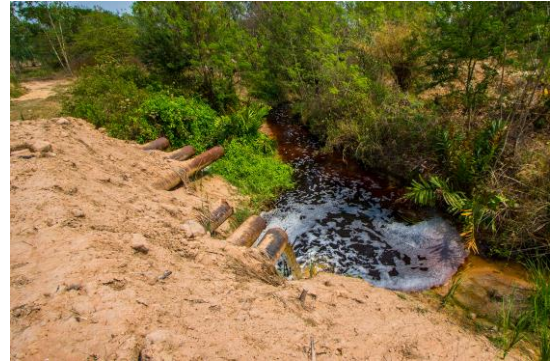
Picture 23: Outflow of wasted water
