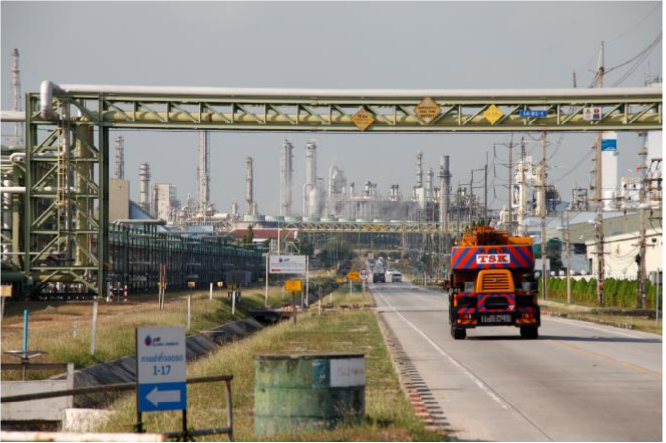
Photo 10: Petrochemical complex in Map Ta Phut. Photo by Ondřej Petrlík, Feb-2016.
