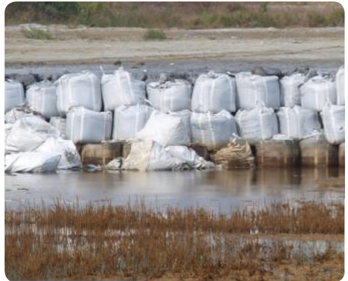
One of the sites where waste incineration fly ash is landfilled in Taiwan.
