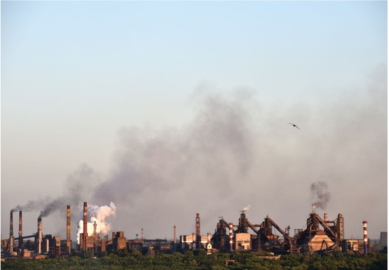
Kryvyi Rih: The city is a coal mining and metallurgy centre of Kryvbas. The biggest polluter of its environment is the global steelworking corporation ArcelorMittal. Photo: Stanislav Krupar / Arnika
