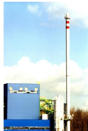
The incinerator with the capacity of 10.000 tons per year consumes 1.134 tons of calcium hydroxide and 140 tons of activated carbon and transforms them into hazardous waste. The contaminated activated carbon is incinerated in the incinerator itself.
