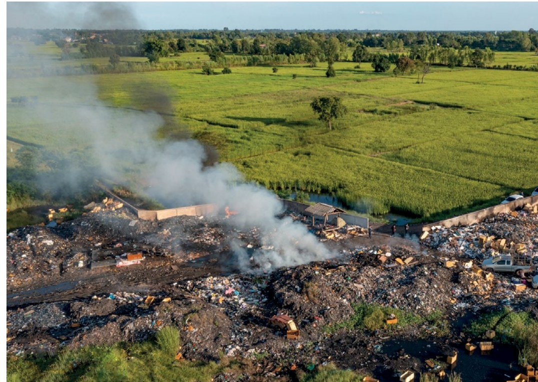
Figure 13: Dumpsite surrounded by rice fields. Photo by © Karnt Thassanaphak, EARTH
