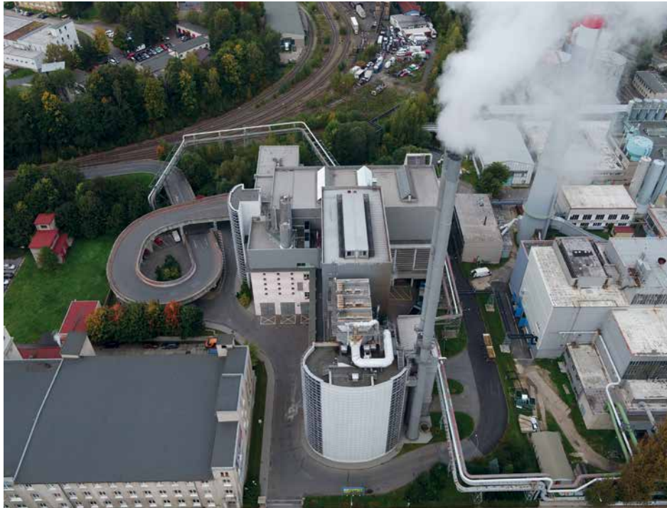
Photo 2.1: Municipal Waste Incinerator (ZEVO) Termizo, a.s. Liberec, as it looked in 2021. Photo taken from a drone by Marek Jehlička (skyworker.cz).
