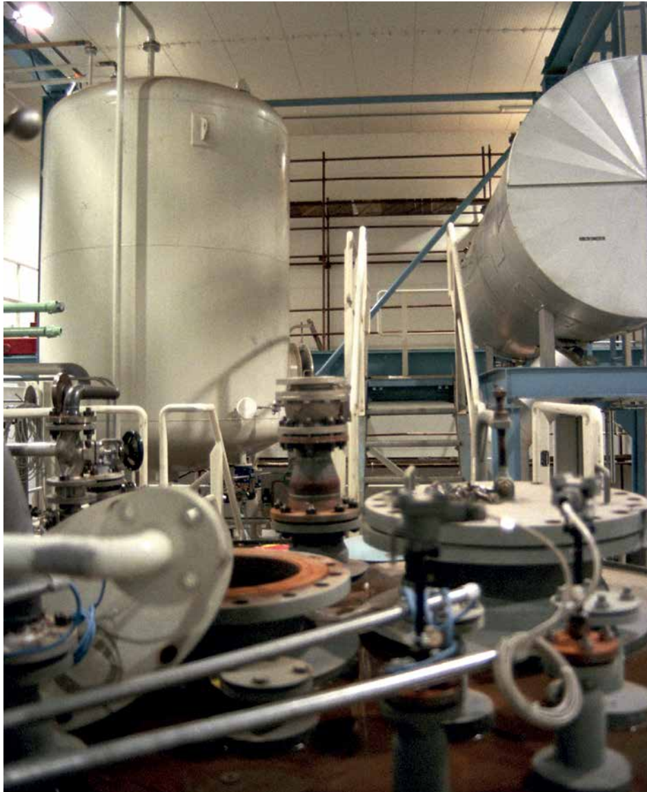
Photo 3.19: Reactor for base catalysed decomposition (BCD) used in Spolana Neratovice, Czech Republic, for dioxin and organochlorine pesticide decomposition. Photo: Jindřich Petrlík, Arnika.
