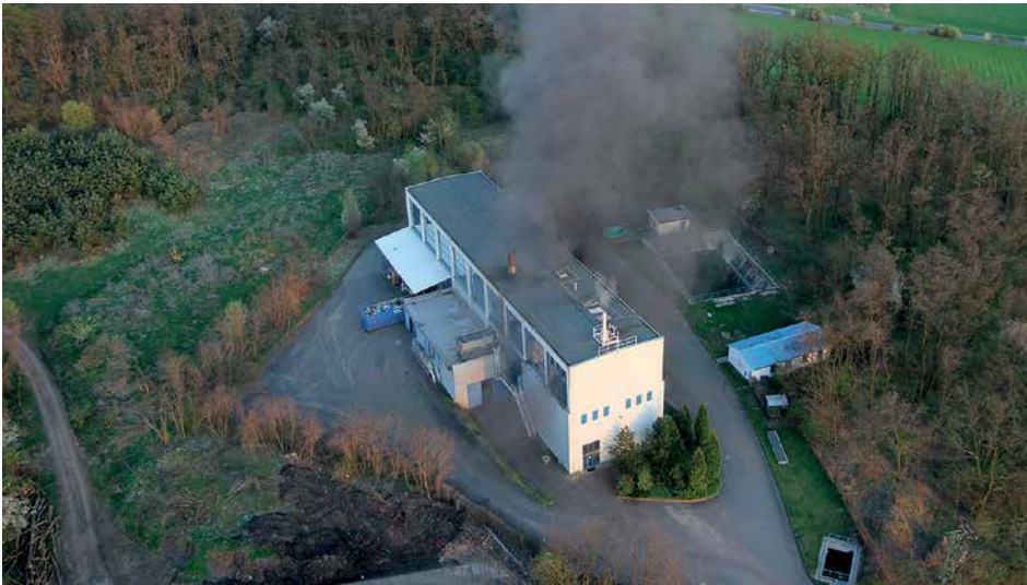
Photo 7.10 A mismatch between incinerator technology and an untested dioxin filter can also lead to an incinerator accident, as happened in April 2013 at the hazardous waste incinerator in Lysá nad Labem (Arnika, 2013). Photo: Arnika archive.
