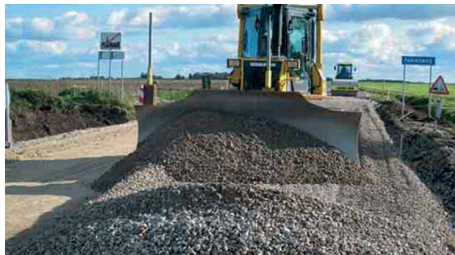
Photo 10.9: Ash and slag from the Iru incineration plant are also used in road construction, as in the Netherlands. Photo: Jäätmed Artiklite arhiiv.
