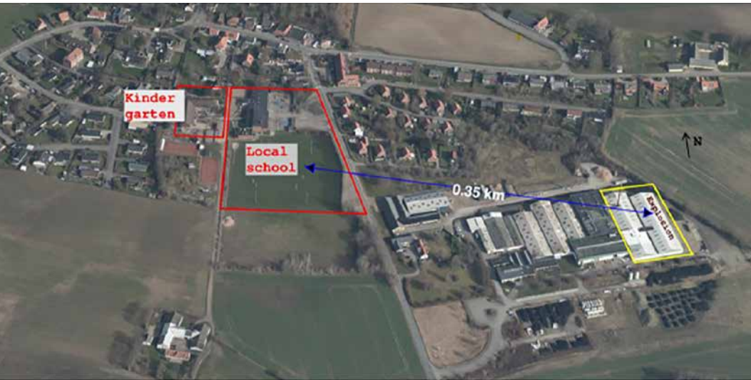
Figure 7.1: Pyrolysis plant located at the outskirts of the Egebjerg rural community. Source: (Hedlund, 2023).
