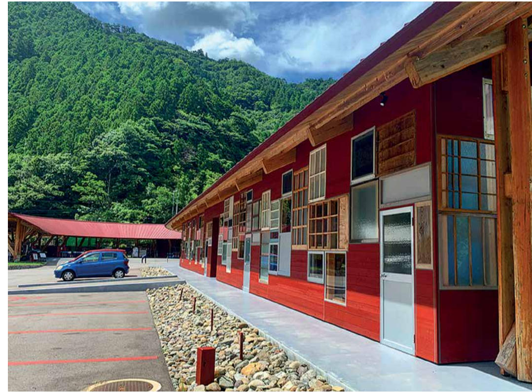
Photo 8.4: Zero-waste management center in Kamikatsu built entirely from materials that were supposed to end up as waste. Photo: Own work (投稿者撮影), CC0, https://commons.wikimedia.org/w/index.php?curid=108202162 .
