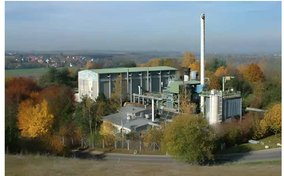
Photo 2.3: Pyrolysis in Burgau, according to Gleis (2012) expensive in construction and operation. Photo: LfU Bayern.
