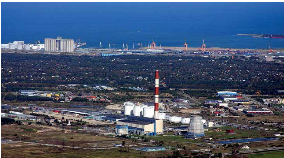
Photo 10.8: The Tallinn WtE in Iru is close to the sea, where waste is imported. Photo: Bjoertvedt – Own work, CC BY-SA 3.0, https://commons.wikimedia.org/w/index.php?curid=9110788 .
