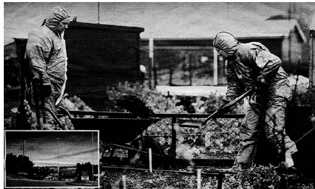
Photo 5.5: A photograph from contemporary press captures the decontamination of the area affected by the use of fly and bottom ash from the Byker incineration plant in Newcastle. Photo: Public Interest Consultants Archive, UK.
