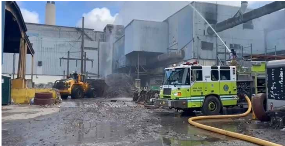
Photo 7.21: Firefighters attempt to extinguish flames at Covanta's Doral trash incineration plant in February 2023. (Source: DeLuca, 2024). Photo: Screenshot from Miami-Dade Fire Rescue video.
