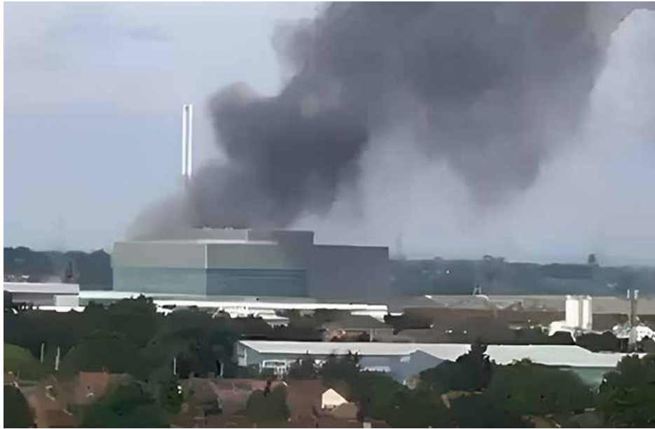
Photo 7.1: Fire in the WtE (Waste-to-Energy) plant in Beddington in July 2019. Photo: London Fire Brigade (@LondonFire).
