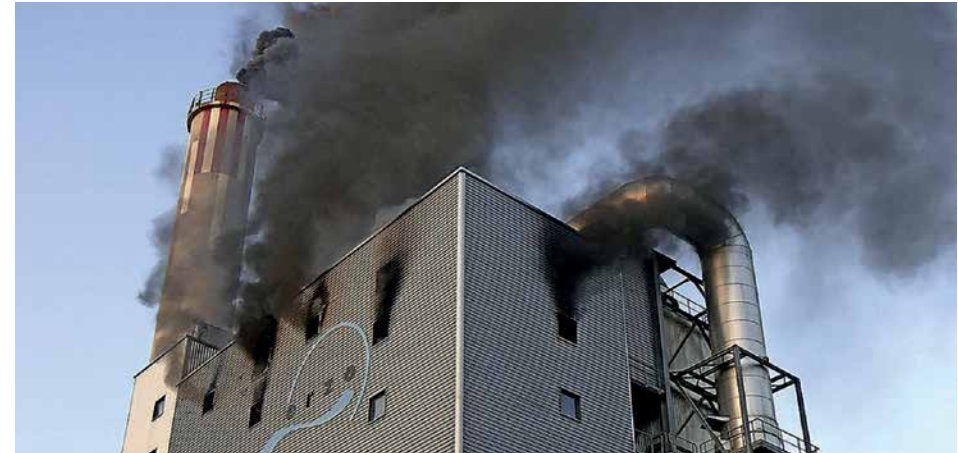
Photo 7.4: A fire at an incinerator in the Aargau canton of Switzerland on May 28, 2015, affected part of the flue gas cleaning system. Black smoke was seen coming from the windows of one of the upper floors (badische-zeitung.de, 2015). Photo: Canton Police, Aargau, Switzerland.
