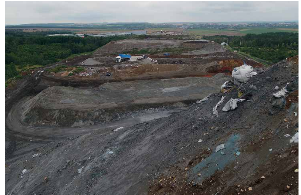
Photo 9.7: The AVE CZ landfill in Benátky nad Jizerou stores bottom ash from WtE Malešice (Prague) in its rear section and uses it, sorted by fractions, for surface treatments. Approximately 70,000 tons of such waste ended up in the landfill in 2018. Photo: Marek Jehlička (skyworker.cz).
