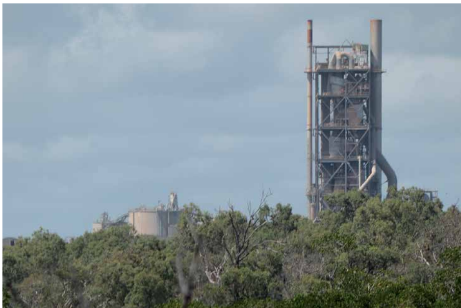
Photo 5.21: The Cement Australia Fisherman's Landing cement plant in Gladstone, Queensland, Australia, experimentally incinerating PFAS-containing firefighting foams, even though it did not reach the minimum target DRE of 99.9999 % for many PFAS compounds, suggesting their release into the atmosphere. Comparing these data with existing literature supports the hypothesis that high temperatures alone are not a guarantee of PFAS destruction in incineration facilities (Kuepou et al., 2022); (Cement Australia, 2017). Photo: Jindřich Petrlík, Arnika.
