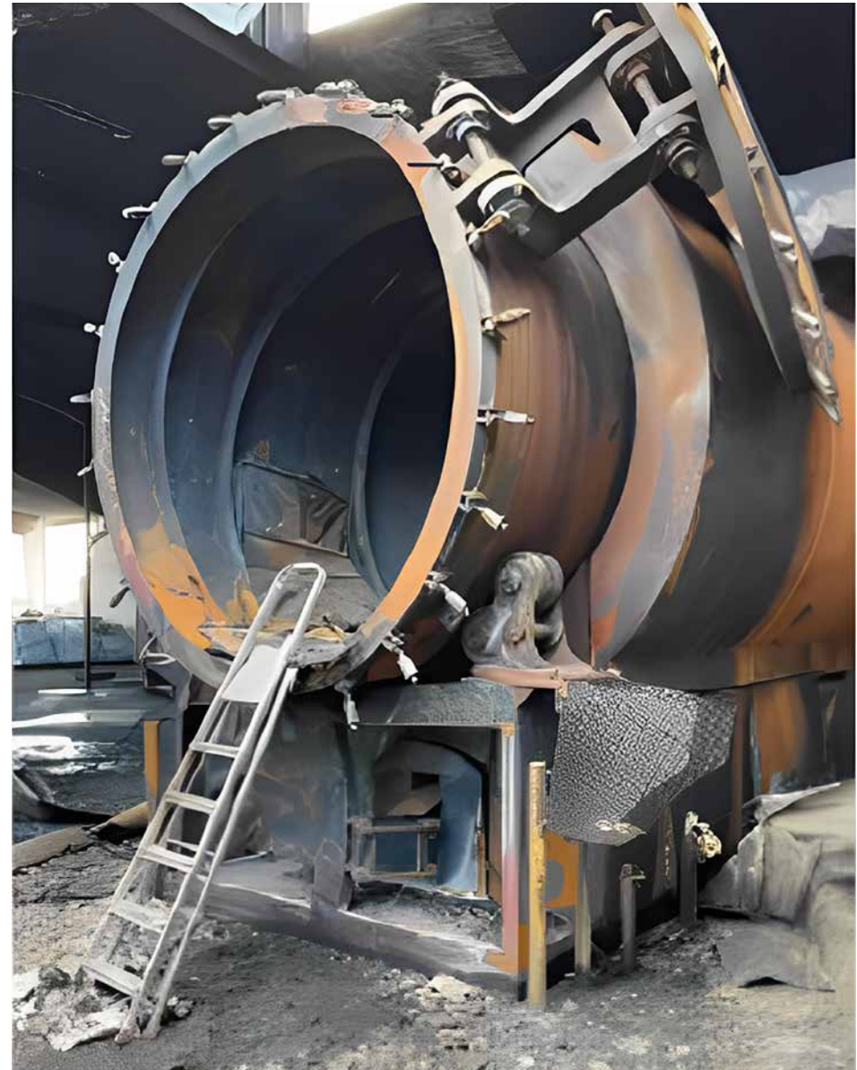
Photo 7.17: Reactor endcamp torn open, deformed (2021). (Source: Hedlund, 2023).
