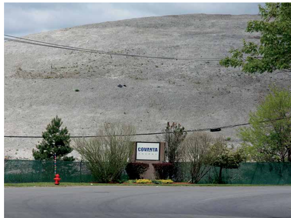
Photo 5.27: Storage of residues from the Covanta incinerator (so-called monofill) in Haverhill, Massachusetts, USA. (Source: Connett, 2013)
