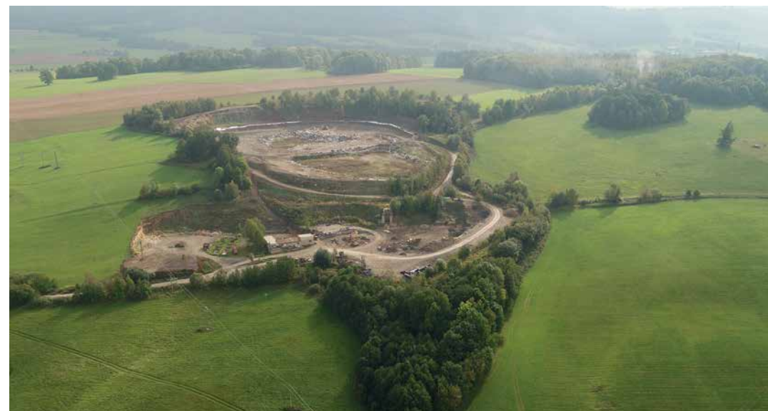
Photo 5.3: When using a mixture of fly ash and bottom ash from waste incineration for surface adjustments on landfills, such as at the Větrov landfill near Frýdlant, Czech Republic (the mixture from WtE Termizo Liberec is used), the specific environmental conditions for leaching dioxins need to be taken into account. A drone photo taken in 2021: Marek Jehlička (skyworker.cz).
