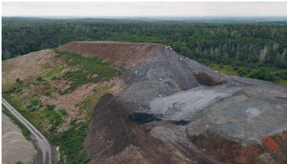
Photo 3.17: Waste mound in the rear part of the landfill in Benátky nad Jizerou, mostly composed of bottom ash from WtE Malešice (Prague). Photo: Marek Jehlička (skyworker.cz).
