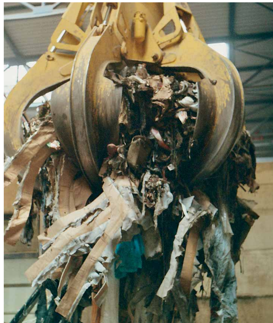
Photo 5.6: Despite their unappealing appearance, approximately 1.5 g TEQ of dioxins enter an incinerator the size of the WtE Malešice (Prague) in municipal waste each year. Far more exits the incinerator. Photo: Jindřich Petrlík, Arnika.
