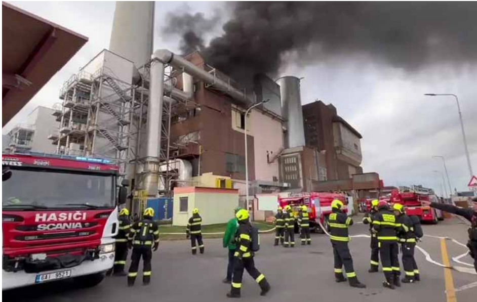
Photo 11.8: WtE plant in Prague – Malešice remained problematic: In October 2021 there was a fire (iDnes, 2023) in technological part (see also Chapter 9.2). Photo: twitter/HasiciPraha.
