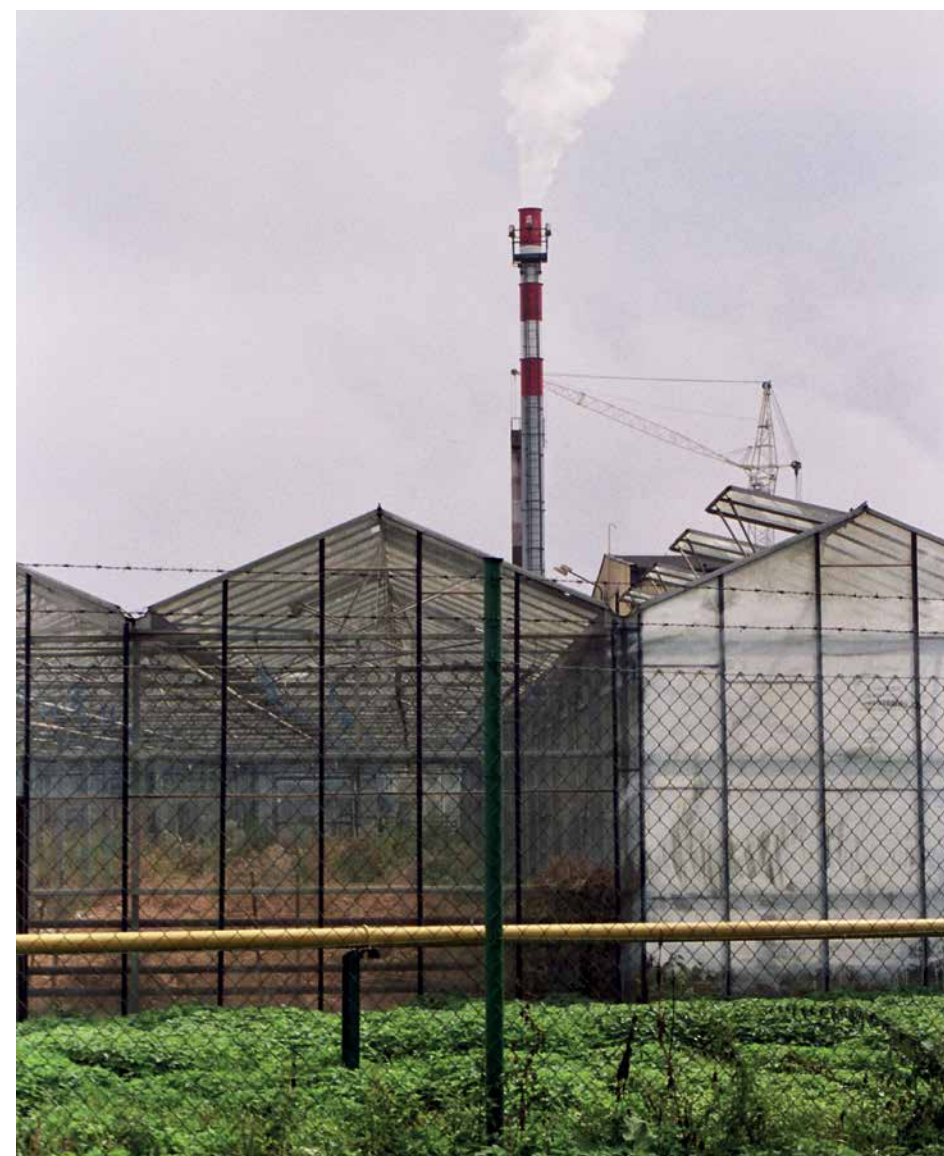
Photo 3.9: The inconspicuous Megawaste incinerator in Prostějov, heating surrounding greenhouses, became the source of a mercury leak in 2003. Photo: Jindřich Petrlík, Arnika.
