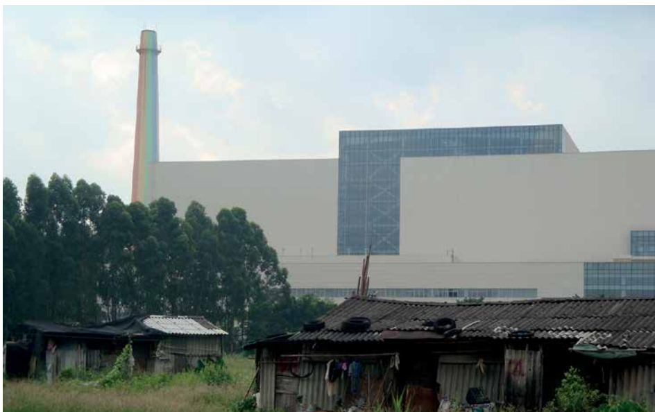
Photo 9.1 Municipal Solid Waste Incinerator in Likeng, China. In China, it is cheapest to build new WtE. Photo: Jitka Straková, Arnika.
