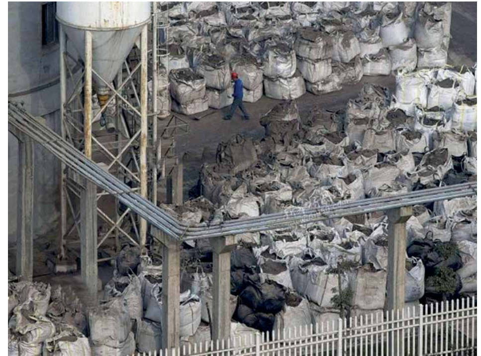
Photo 3.7: Ash stored in the yard of a municipal waste incinerator in Wuhan, China—likely a source of fugitive dioxin emissions. (Source: Zhang et al., 2015)
