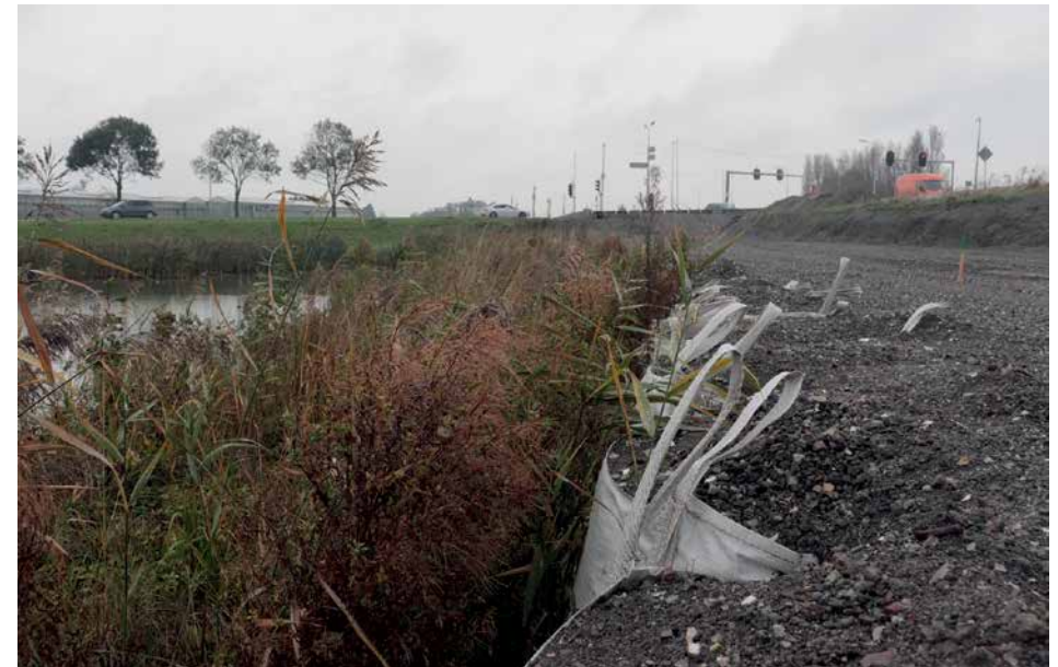
Photo 3.27: Incineration ash is widely used in the Netherlands, as visible in the terrain modifications in Katwijk aan Zee. Photo: Jindřich Petrlík, Arnika.
