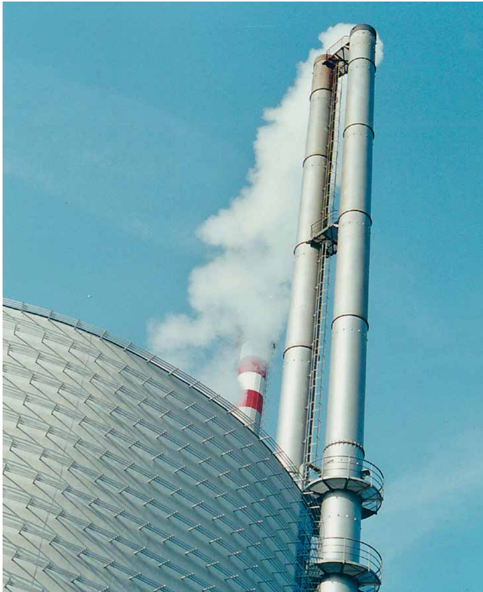
Photo 5.1: WtE Termizo Liberec (Czech Republic) initially failed to meet the 0.1 \text{ ng TEQ}\cdot\text{m}^{-3} limit for dioxins, thus requiring the costly addition of a filter (see Chapter 9.1.1). Photo: Jindřich Petrlík.
