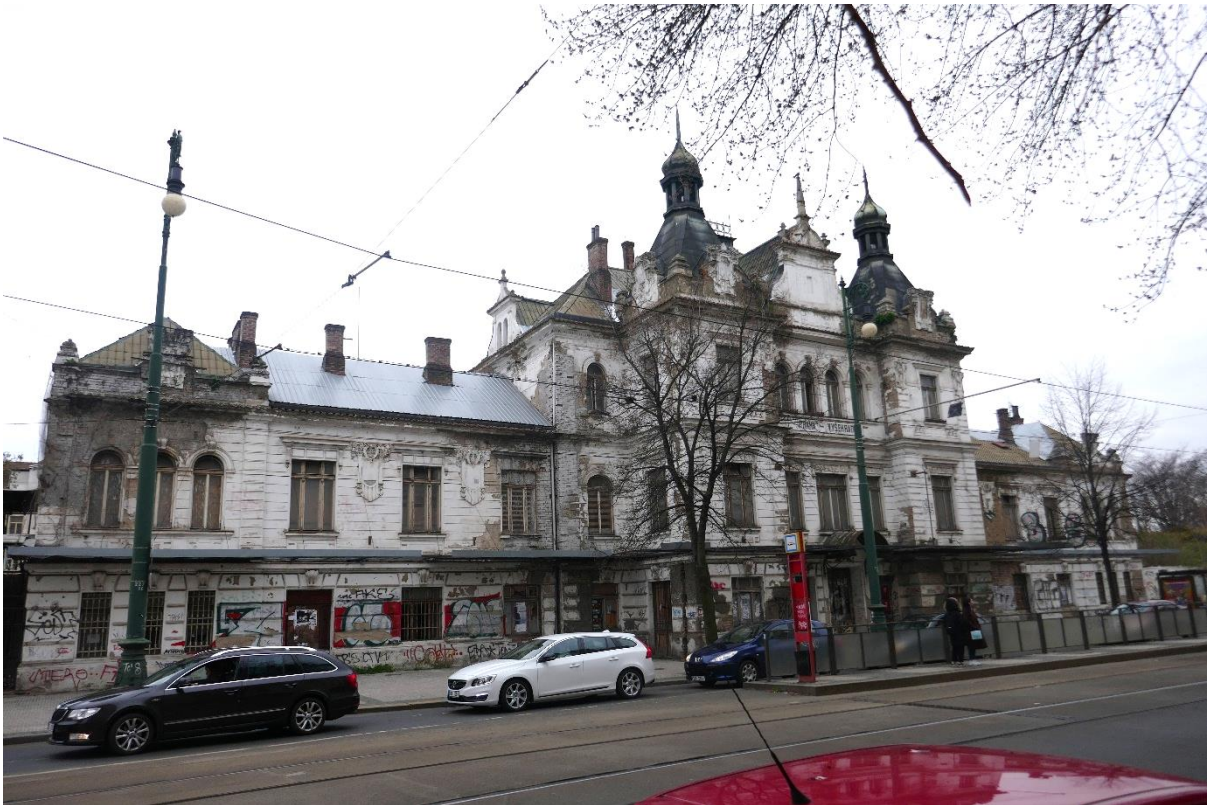
Fig 20 Vyšehrad Station, March 2019.
