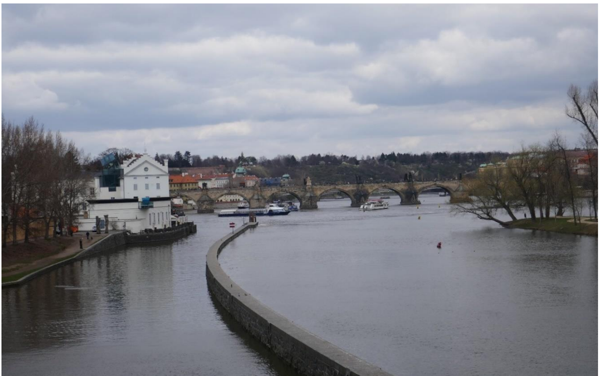
Fig 6 The entry channel to Smíchov Lock looking north (downriver) from the Legion Bridge; the outer wall would leave the existing one and swing further out to create the new channel; Charles Bridge in the background, tourist boats circling in front of it.
