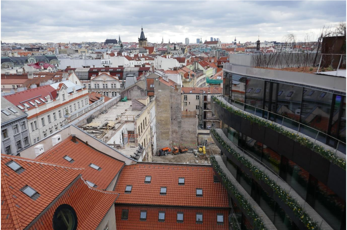
Fig 28 Old and new looking south-east from the roof of the new building.
