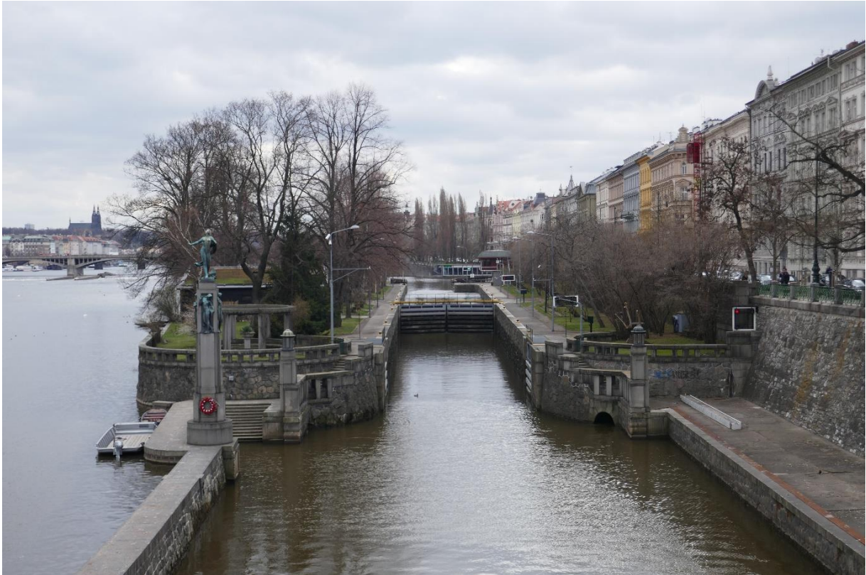
Fig 5 Smíchov Lock looking south (upriver) from the Legion Bridge; the second basin would be on the outside of the walled island, with a low wall between the river and the channel similar in scale to that in the left foreground.
